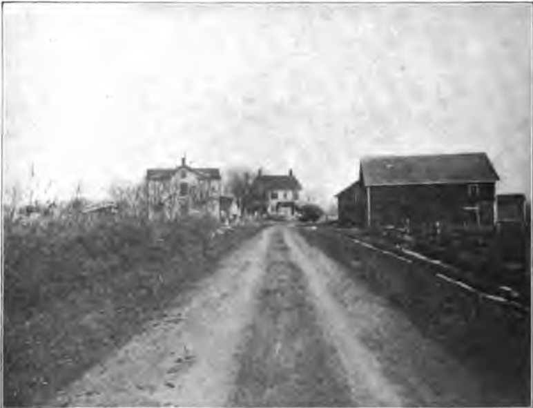
Neshanic road, Somerset Co., after improvement.
